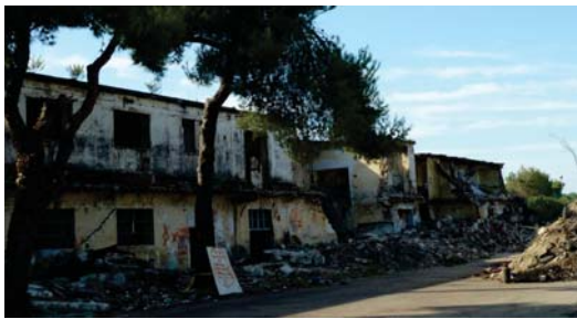
Fig. 11 Ex-American collapsed hospital, Calambrone, Italy
