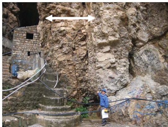
Fig. 5 Fractured zone of CBF
