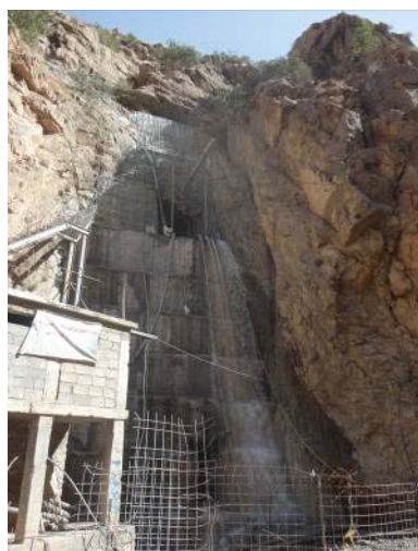
(b) After plugging
