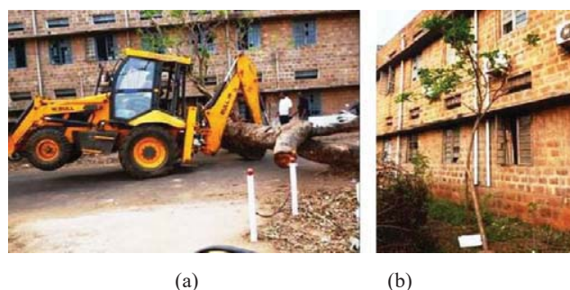
Fig. 19 (a) Removal of debris of fallen trees at Andhra University (b) A restored Phyllanthus embilica tree in the Botany Department at Andhra University Campus
