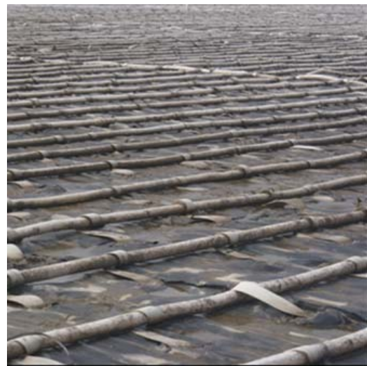
Fig. 4 Plastic pipes laid horizontally for water discharge and to support the membranes
