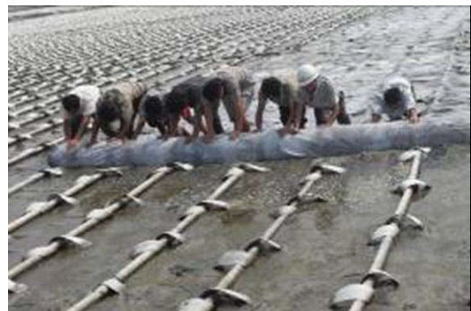
Fig. 7 Working photo of laying vacuum membrane
