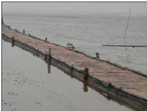
Fig. 3 Complete floating bridge
