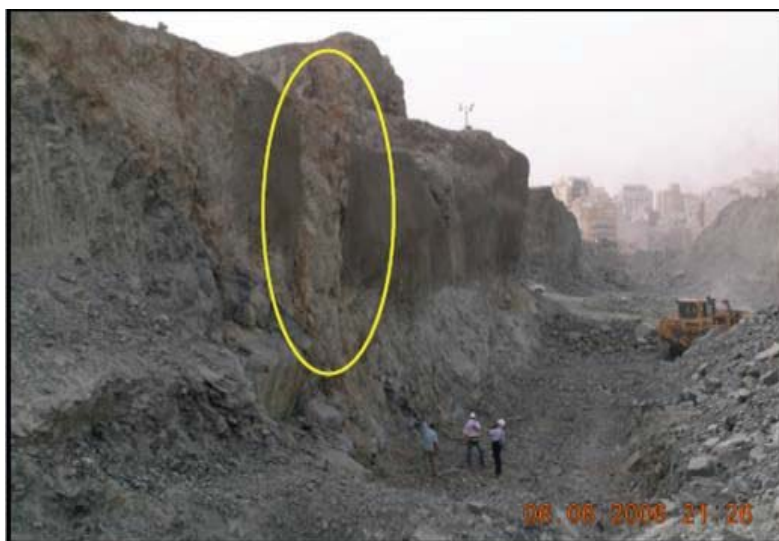
Fig. 2 View of the site condition of the site, the yellow circle indication the failure section
