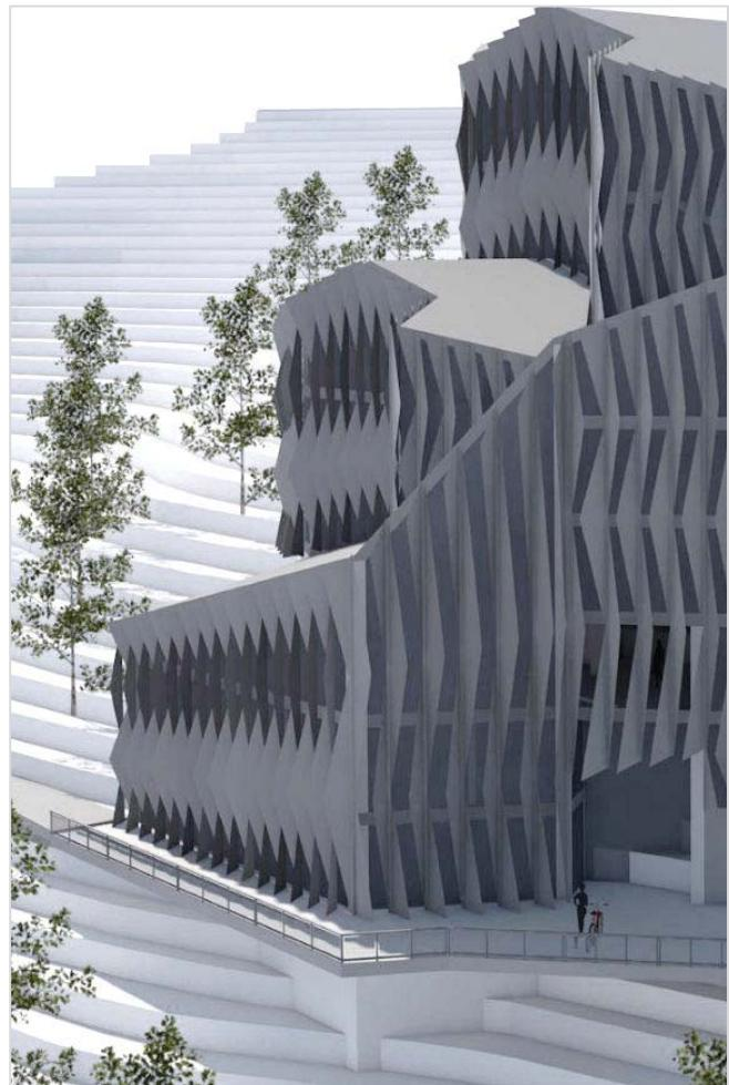
Fig. 26 Triangular flectofin-elements in upright arrangement [8]
