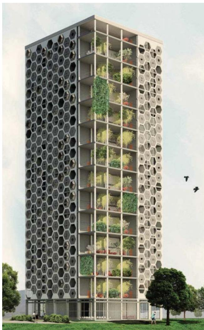
Fig. 20 Honeycomb-façade, elements partially opened + partially closed [11]
