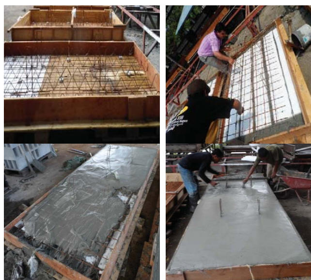
Fig. 3 Preparation, fabrication, and casting of PFCSP specimens
