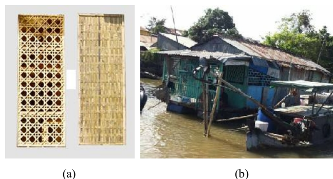
Fig. 11 The façade of floating houses are made of wickerwork, latticework, and reed weaves. (a) [12], (b) [6]
