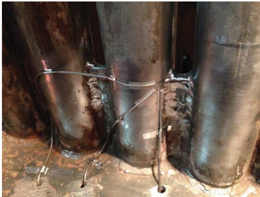
Fig. 3 Strain gage installation on boiler tubes
