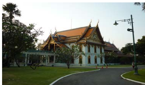
Fig. 2 The traditional Thai style building [2]
