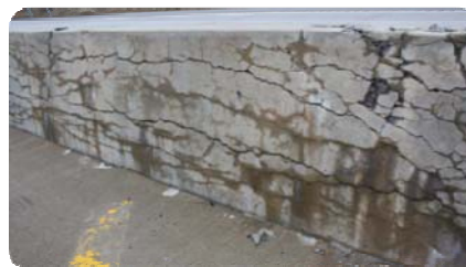
Fig. 5 Deterioration in Arkansas Highway Projects
