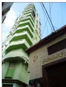
Fig. 6 High rise residential building in Sayied Darwish Street
