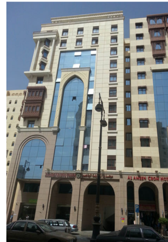
Fig. 3 Front view of the case study building in Madinah
