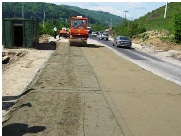
Fig. 1 Roller compacting
