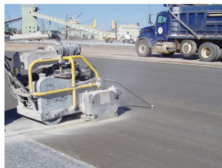
Fig. 3 Transvers joint
