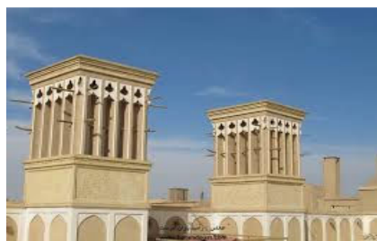
Fig.1 Wind catchers that have more than one side facing the prevailing wind
