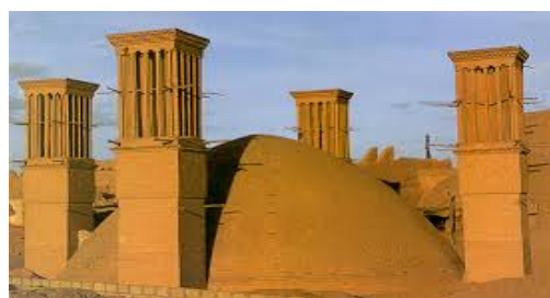
Fig. 6 A water reservoir and wind catchers around it
