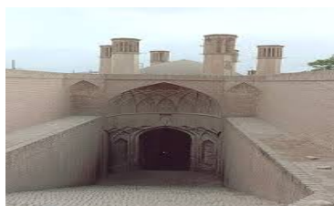
Fig. 5 The entrance of a water reservoir toward the storage tank
