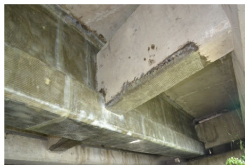
Fig. 1 Strengthening of Bridge Girder
