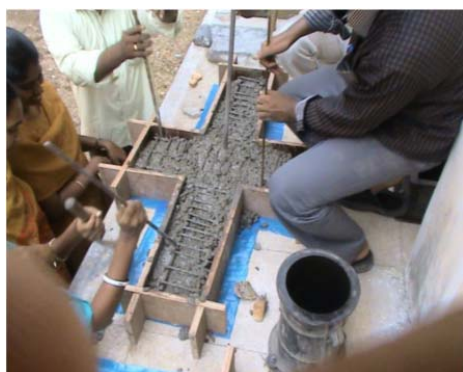
Fig. 9 Casting of beam column joint
