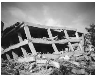
Fig. 5 Beam column Joint failure
