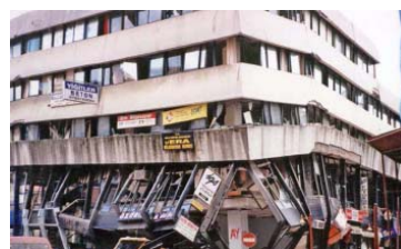
Fig. 1 A seriously damaged RC building in Marmara region [2]
