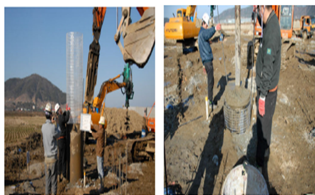
Fig. 6 Construction GESC at the site
