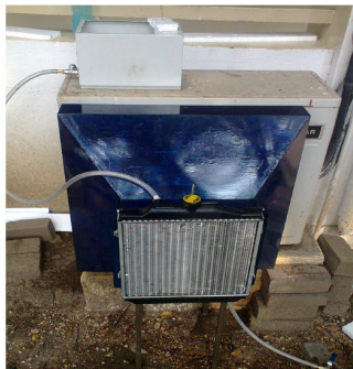
Fig. 1 Experimental set up for the waste heat energy recovery system
