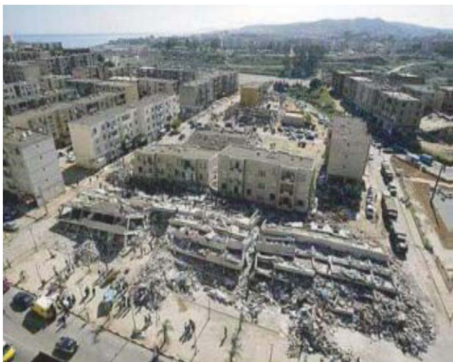
Fig. 2 Building damages observed in the city of Boumerdes (photo from CSEM-EMSC September 2003)
