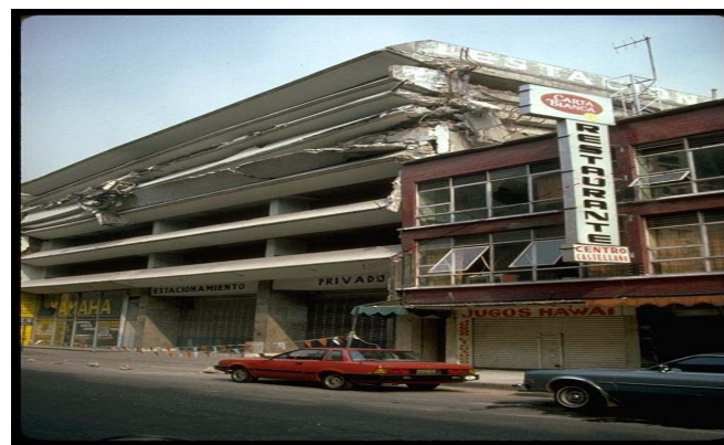
Fig. 1 Buildings have undergone a whiplash during Mexico 1985 earthquake
