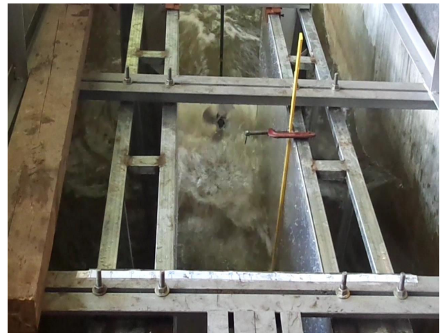
Fig. 6 Turbine placed at the tunnel end
