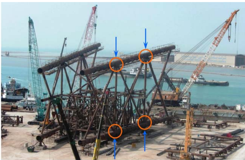
(a) Tubular KT-joints in a jacket structure during fabrication
