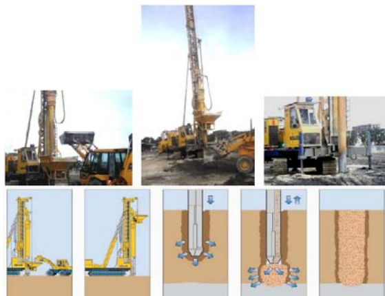
Fig. 1 Bottom-Feed method of stone column construction [5]
