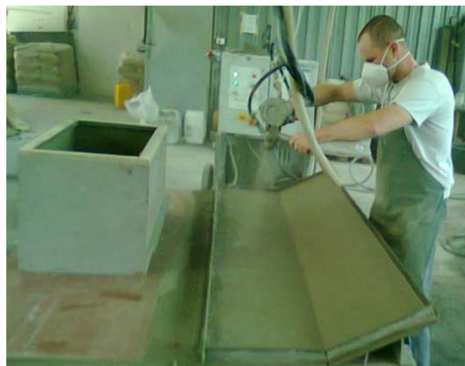
Fig. 3 Spraying of bridge cladding element
