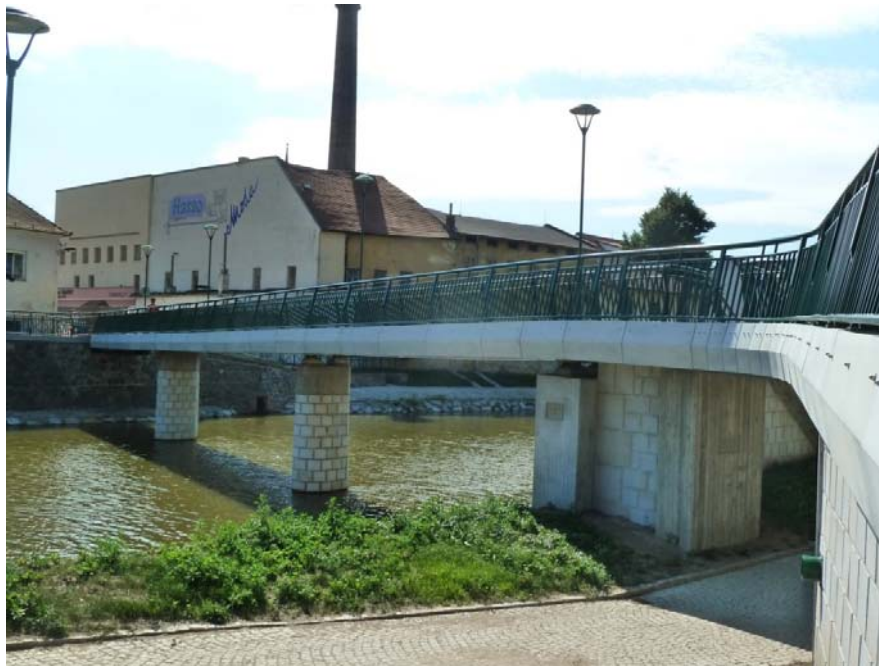
Fig. 4 Bridge cladding elements assembled at the foot bridge across a river
