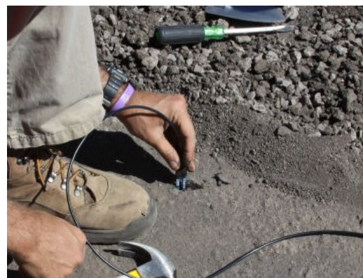
Fig. 3 Installation of a moisture probe
