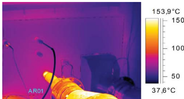
Fig. 8 Combustion Chamber – Right (Air Preheater) Side
