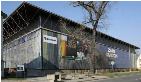
Fig. 12 Roof structure of winter sports stadium in Olomouc city
