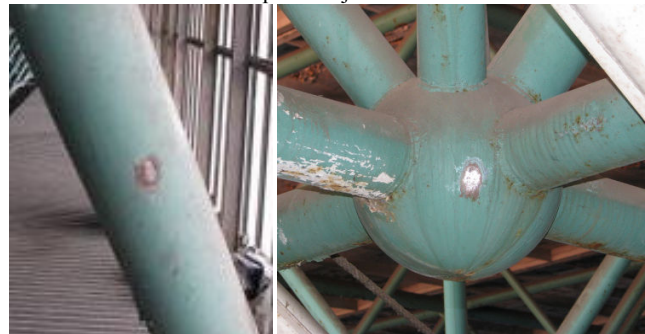
Fig. 15 Illustration of structural members with tested locations prepared for subsequent measuring
