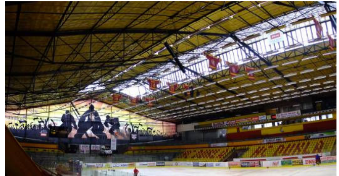
Fig. 10 Roof structure of winter sports stadium in Jihlava city
