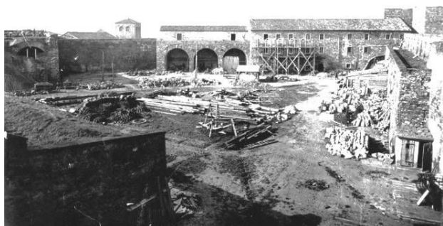
Fig. 3 San Giusto Castle in Trieste: 1930s restoration works
