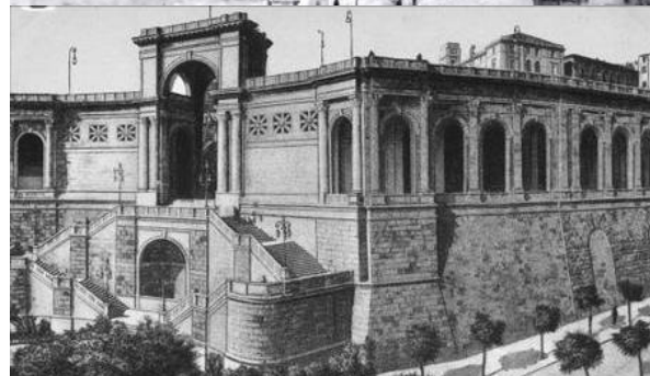
Fig. 6 Cagliari, southern bastions at the end of 19th century: structures built against the walls are clearly visible. They were later removed to build the Bastion of San Remy
