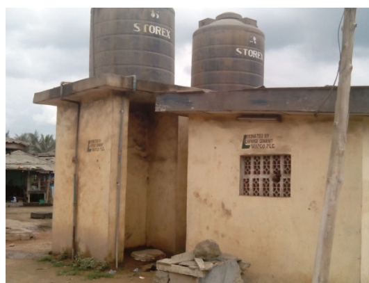
Fig. 6 Abandoned borehole due to contamination from Limestone
