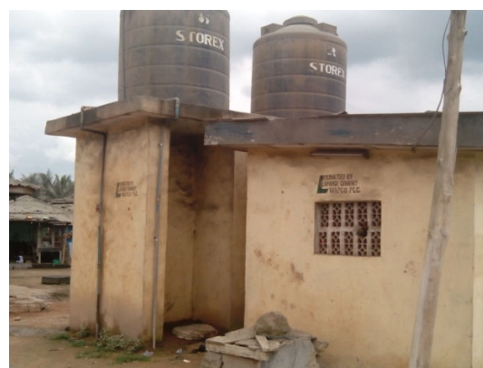
Fig. 6 Abandoned borehole due to contamination from Limestone
