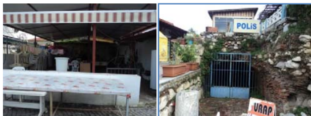
Fig. 6 Important historical buildings in bad condition
