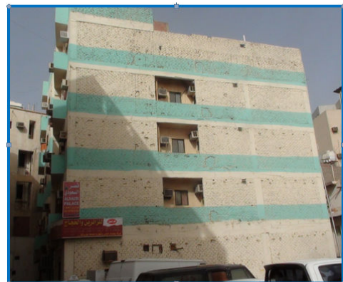
Fig. 6 View of the Case Study Building in Madinah
