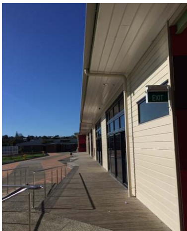
Fig. 3 One-story building with light rain screen wall
