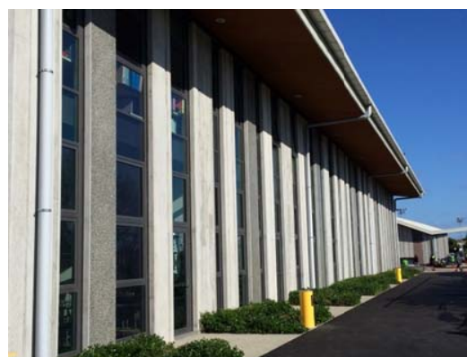
Fig. 1 Maths Building with precast insulated concrete panel walls
