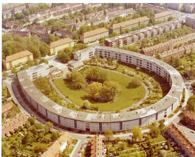
Fig. 2 Hufeisensiedlung in Berlin, built between 1925 to 1933 (one of the first social housing in Germany)
